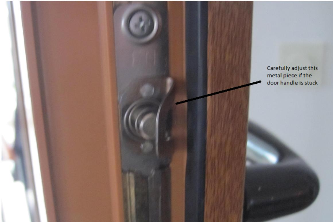
Carefully adjust this metal piece if the door handle is stuck
